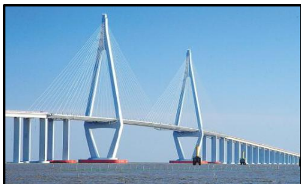
Hangzhou Bay Bridge with ZEFFLE Topcoat: Opened in 2008 (36 km)
