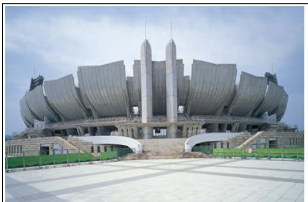
Nagano Olympic Stadium with ZEFFLE Topcoat: Completed in 1996
