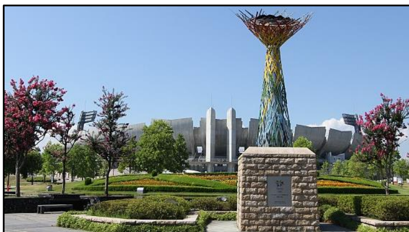
Nagano Olympic Stadium with ZEFFLE Topcoat: Completed in 1996
